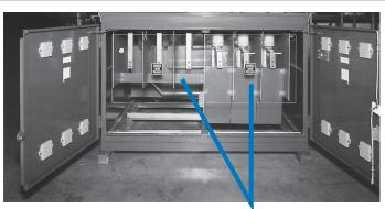
Low-Profile Switchgear Cabinet – Interphase and end barriers are fabricated from Grade UTR Laminate.
